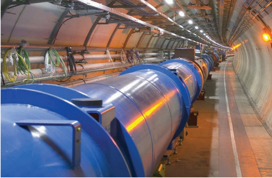
Plate 1 LHC tunnel and beam line. The blue cylinders contain dipole magnets and the liquid helium system required to cool them to superconducting temperatures. (Reproduced by permission of CERN.)
